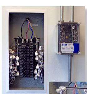
Right: The PowerScout is line powered and the broadband power supply accommodates voltages from 80-600VAC. Left: The PowerScout 24 can use up to 24 CTs to measure any combination single or three-phase loads. Mix and match any of DENT's RoCoil or Split core CTs to monitor building mains and smaller loads simultaneously with a
